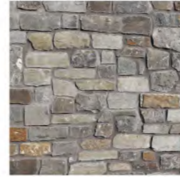
EW07 - Coursed rubble stone slip attached to backing block Black Mountain
