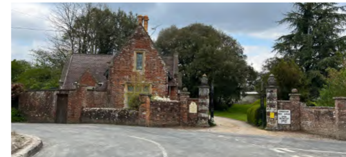
Street View 1, Edmondsham gateway building
